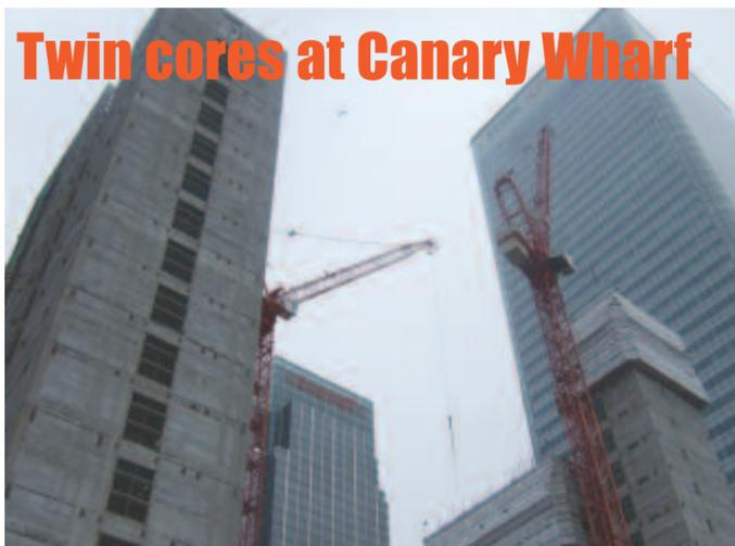
**We have reached a peak with the slipforming of twin cores for the DS3 development at Canary Wharf.**
